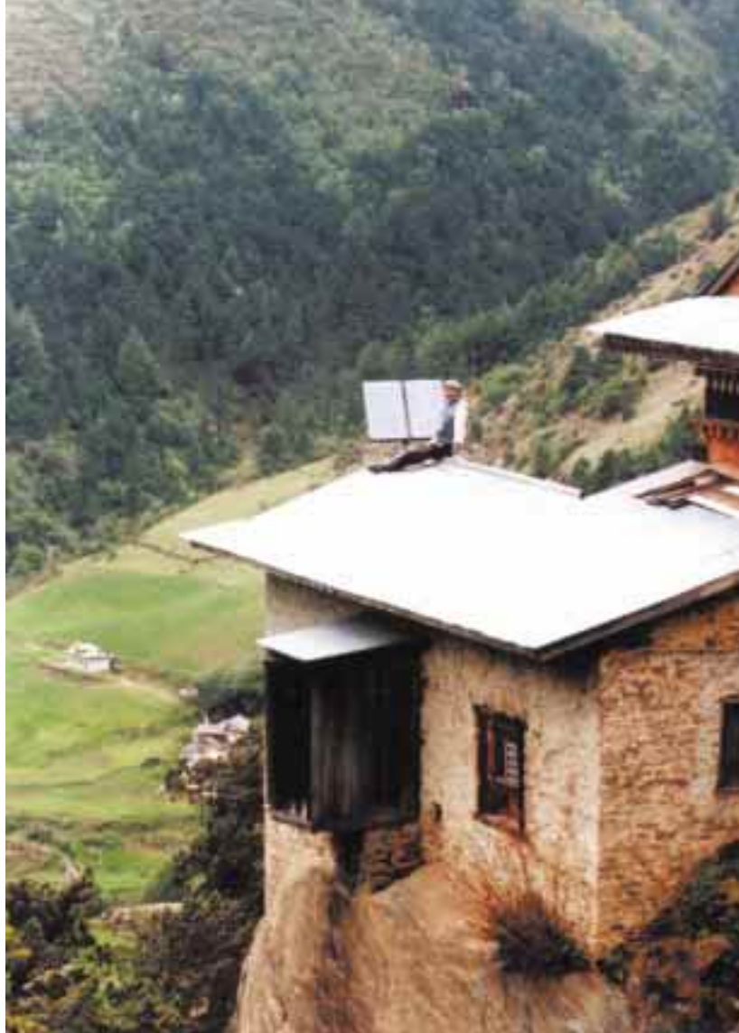
Above: The 150 foot drop made installing the PVs exciting for Dennis.
