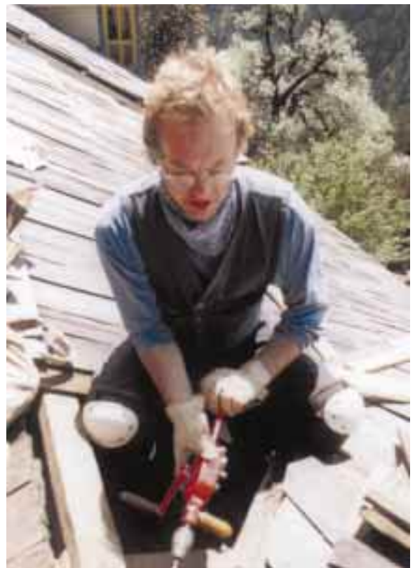
Below: Dennis drilled holes to run the wiring from the roof to the rooms below.
