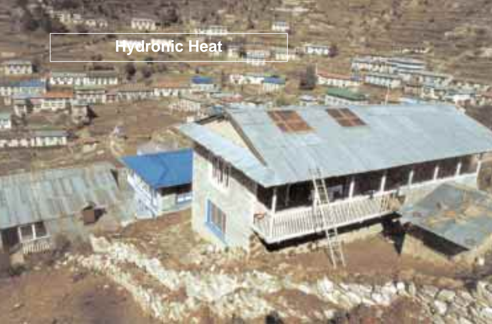
The Namche Bazaar dental clinic, overlooking town. New skylights add natural light and solar gain.
