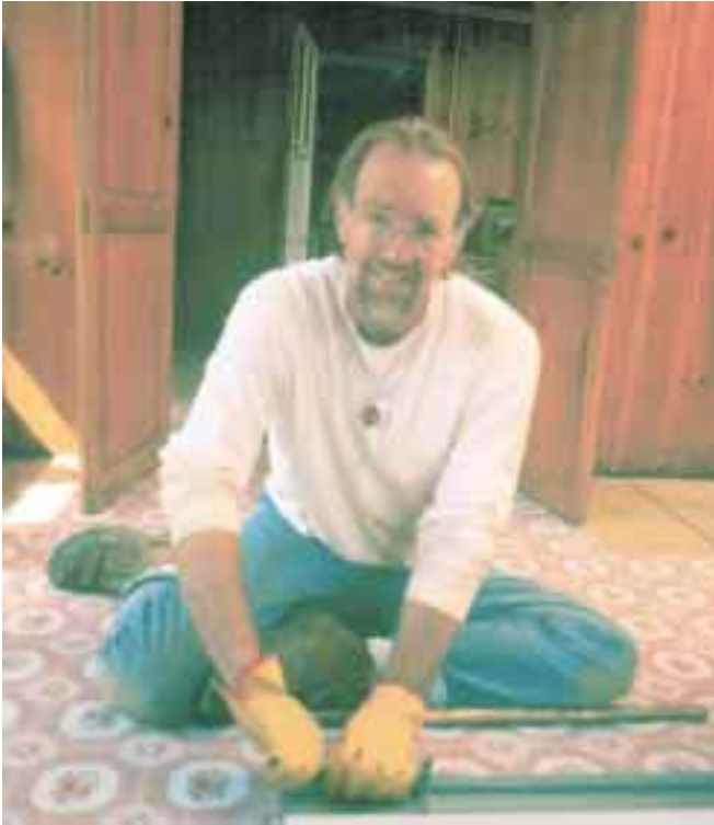
Author Dennis Ramsey with plumbing in progress.
